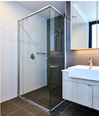
SHOWER SCREEN 2000mm high semi-framed with pivot door and clear laminated glass.
