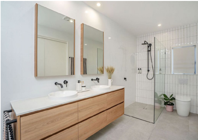
WET AREA CERAMIC TILING WALL TILES AND BATH HOB - Ceramic wall tiles from Begin with Precision colour board schemes to areas as per standard working drawing. Plain aluminium L-shape angle trim to bath hob/riser junction. SKIRTING TILES - 100mm high, from Begin with Precision internal colour board schemes ceramic floor or wall tiles to laundry, bathroom, ensuite, powder room(s) and WC as per standard working drawing.
