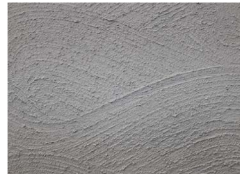
BAGGED BRICKWORK TO SIDES AND REAR *Image is for illustrative purposes only for texture visualisation
